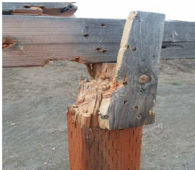
Example of Post Damage
